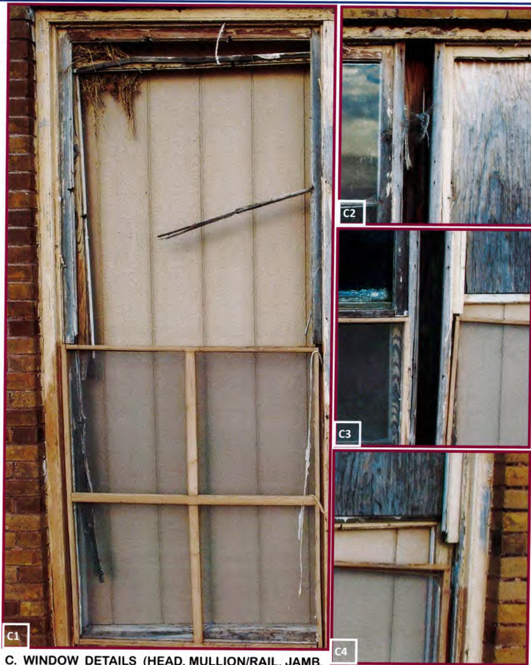
C. WINDOW DETAILS (HEAD, MULLION/RAIL, JAMB,
