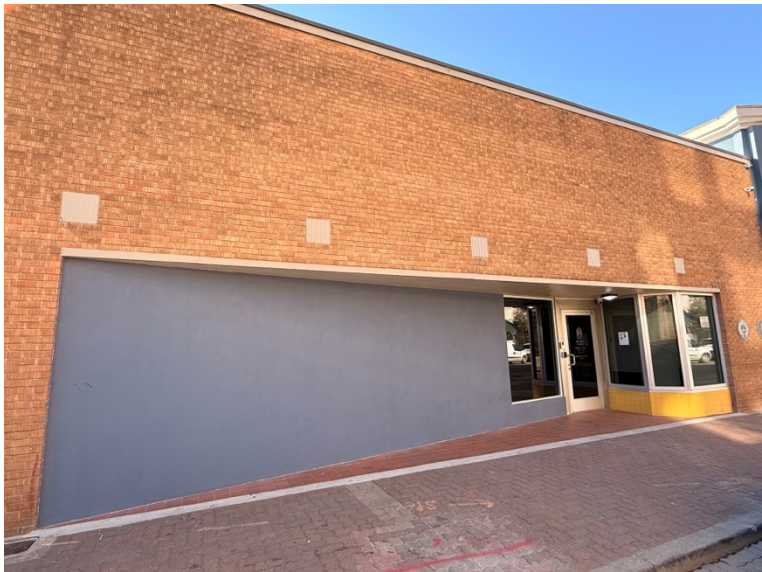
Existing façade after modifications
