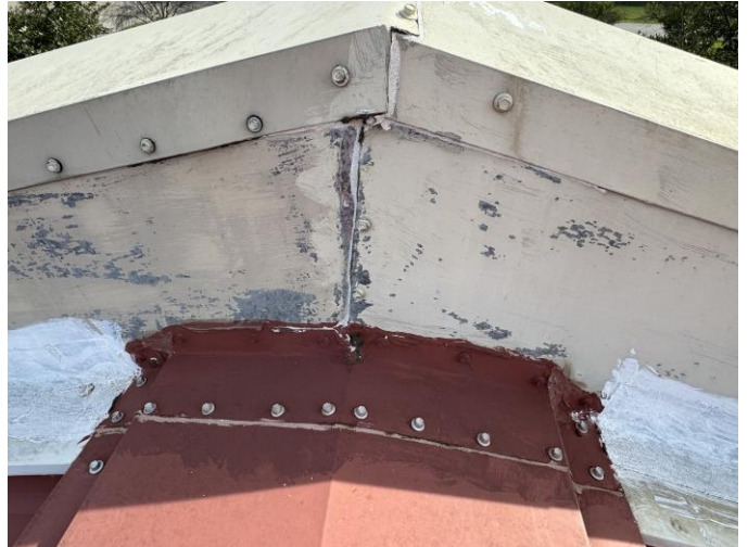
Open holes at wall intersection.
