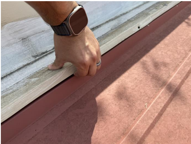
Poorly fastened flashing at wall intersection.
