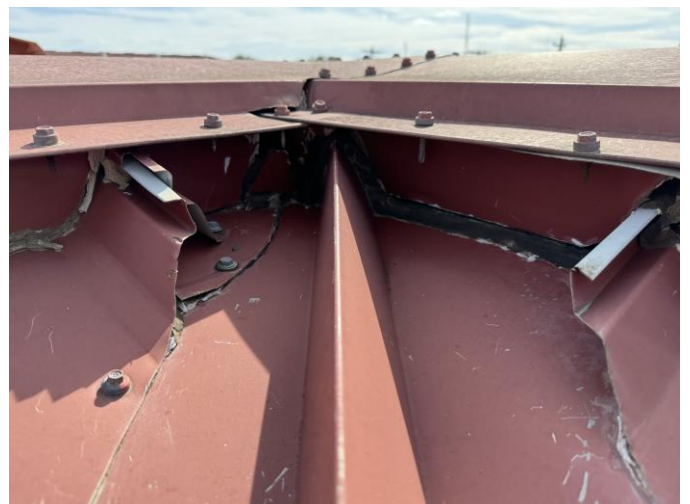
Open holes at laps and corners.
