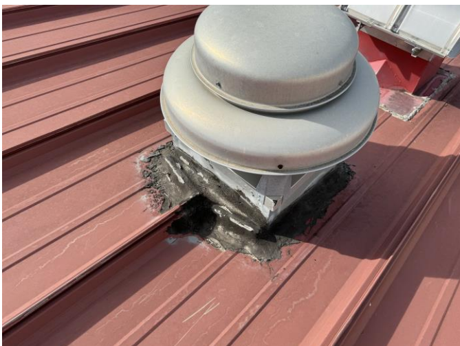
Repairs at roof vent location.
