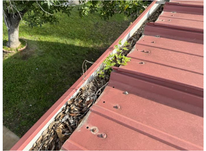
Trash and debris in gutter.
