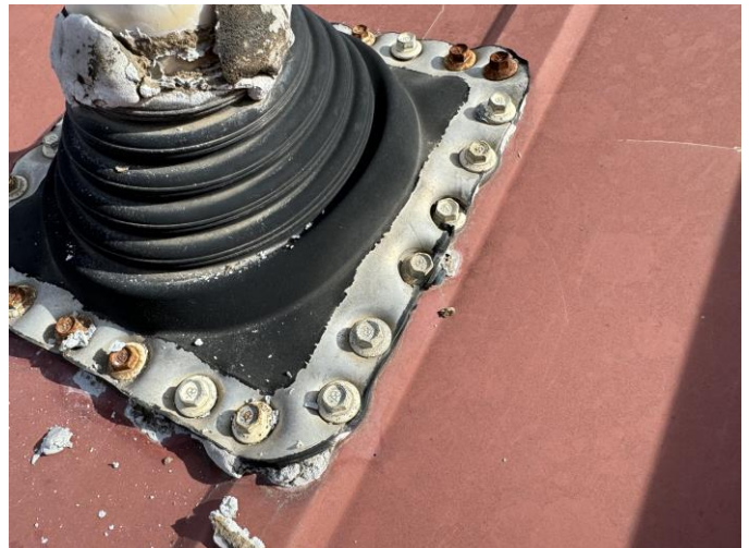
Vent pipe boot in poor condition.
