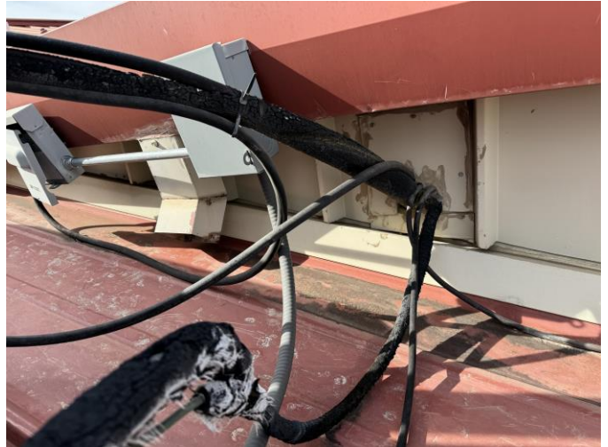
Electrical mounted to gutter.
