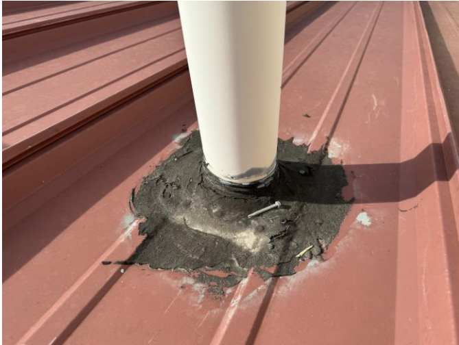
Poor flashing at pipe penetration.
