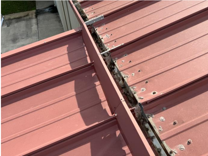
Trash and debris in gutter at roof transition.
