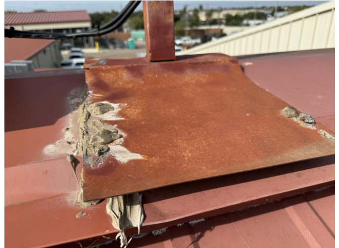
Poor flashing at ridge cap.
