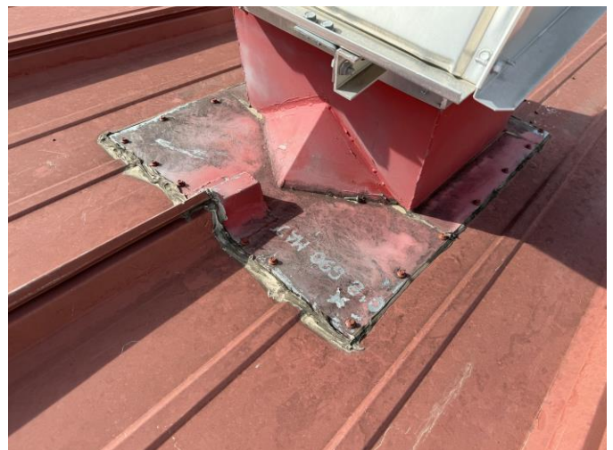
Repairs at vent locations.
