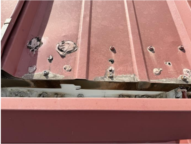
Multiple repairs or fastener holes at eave.
