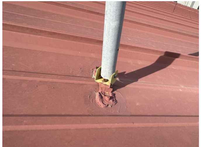
Missing flashing at pipe penetration.
