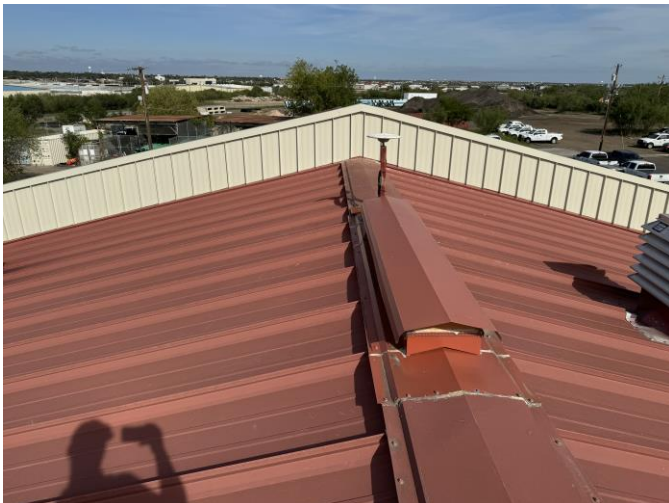
Rooftop vent locations are typical leak locations.
