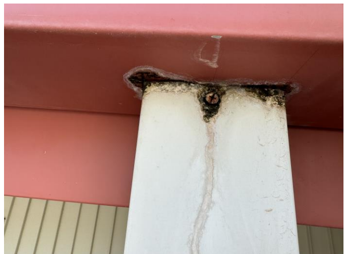
Corrosion at downspout connection.
