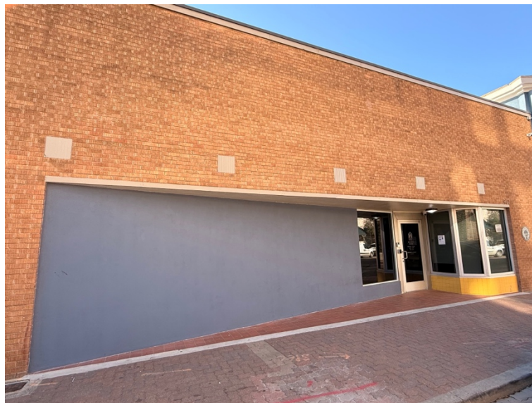
Existing façade after modifications
