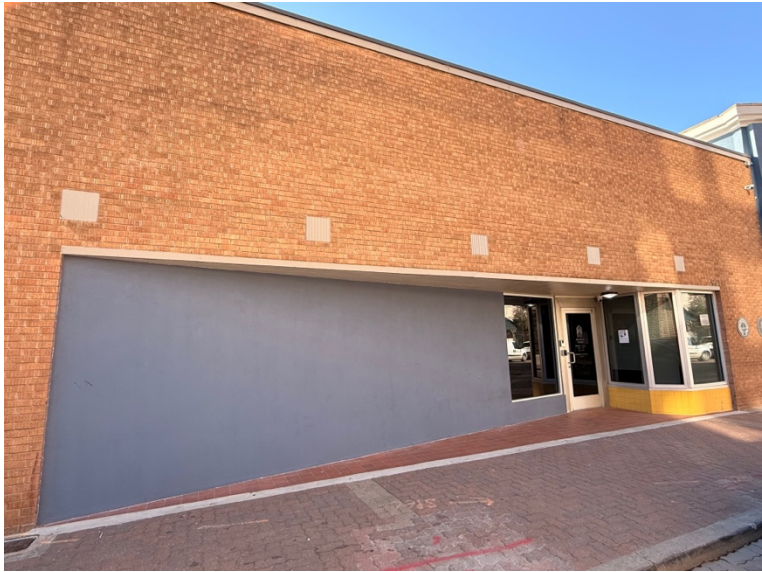
Existing façade after modifications
