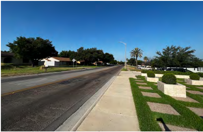
Segment 2: North curb
