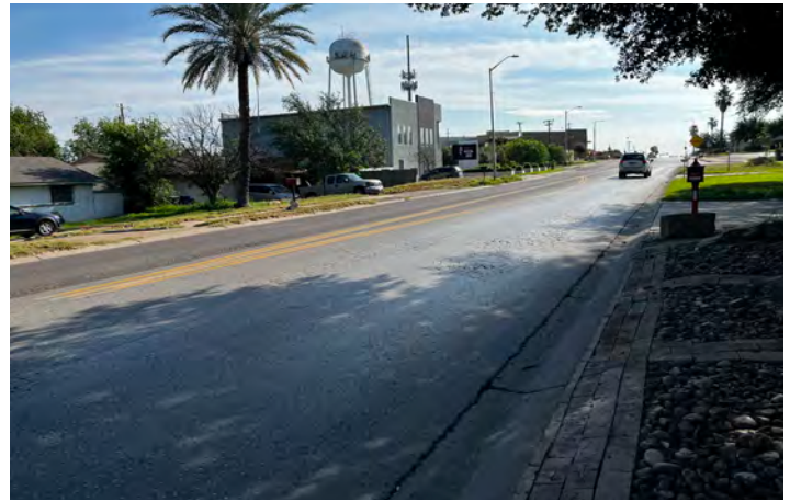
Segment 2: South curb
