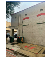
Actual View Condition on Elevation
