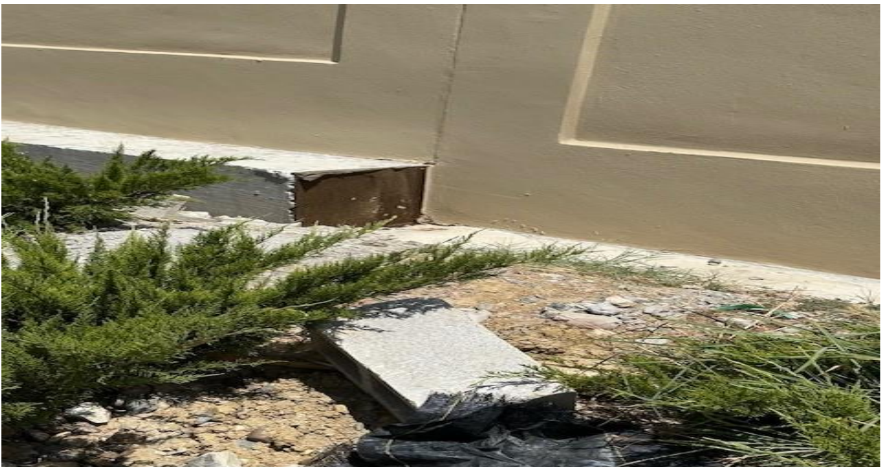
Photo 8: CMU block and expansion board needs to be removed.
