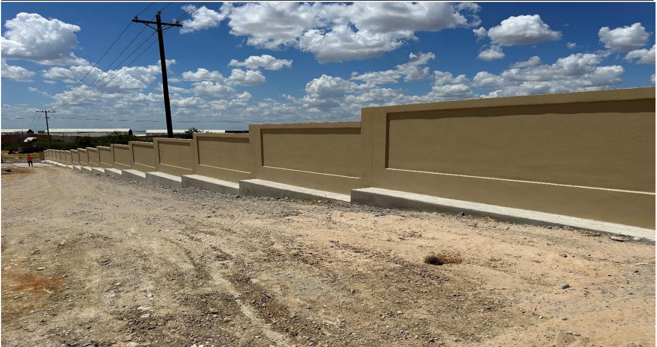
Photo 4 : Grading and CMU Wall has been painted to match existing paint color.
