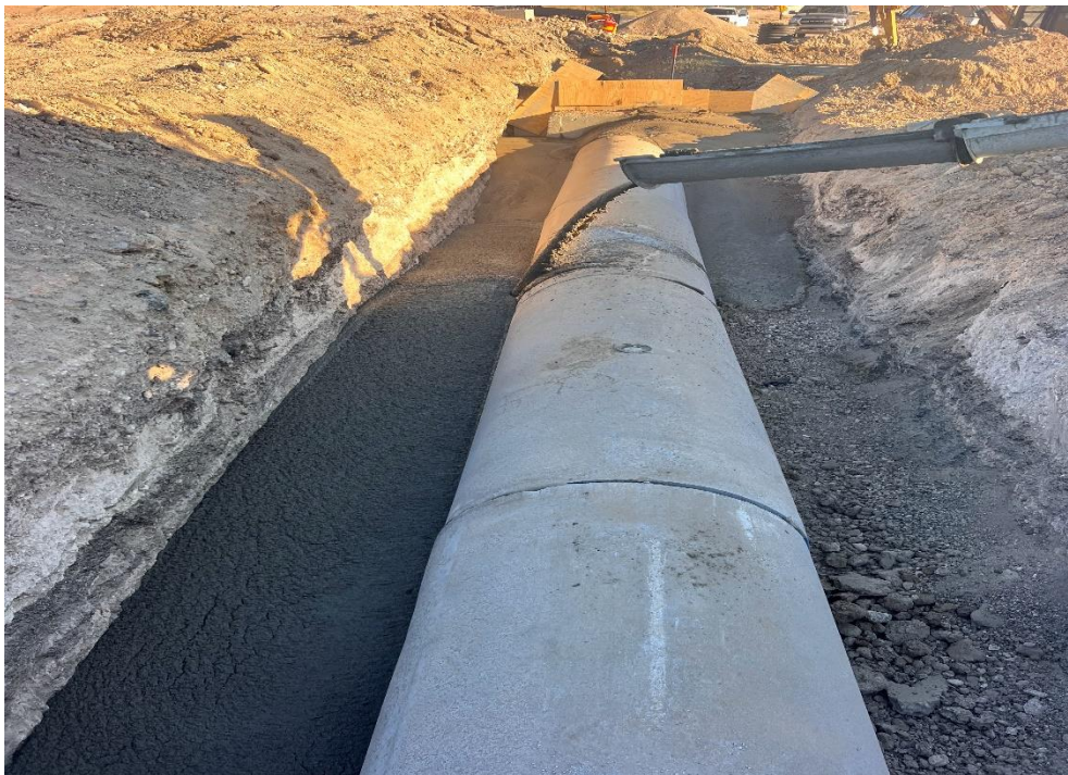
Backfilling pipe with flowable fill
