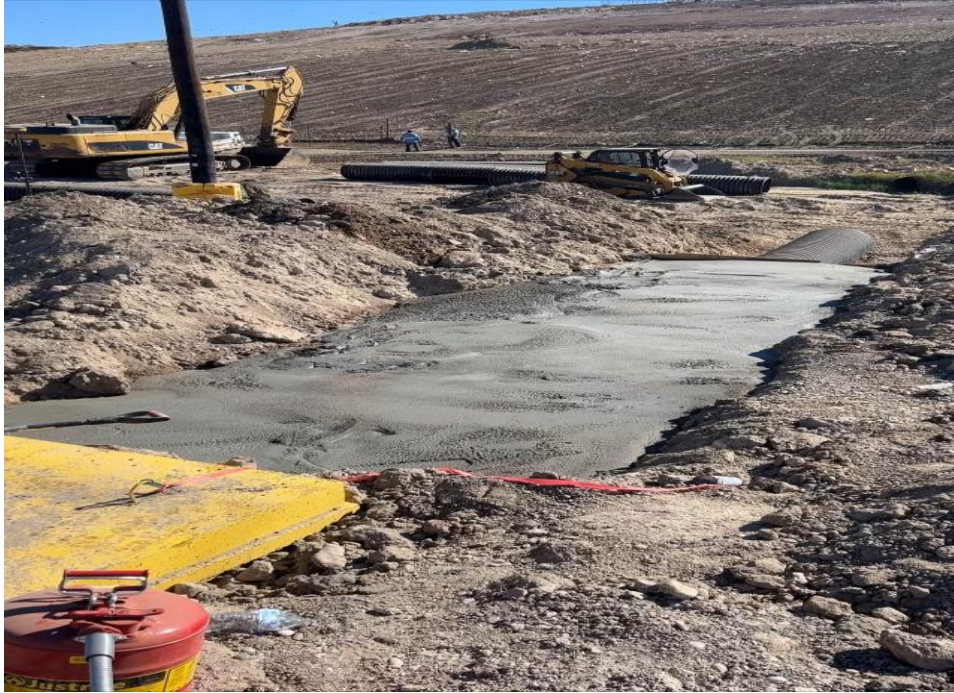
Completed flowable fill over pipe
