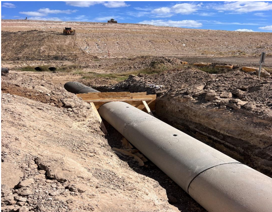
Pipe replacement and new Concrete Pipe
