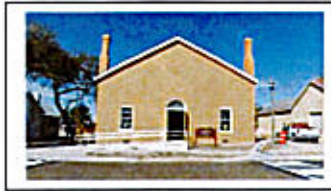
P-24 Former Commissary Environmental Abatement 2010
