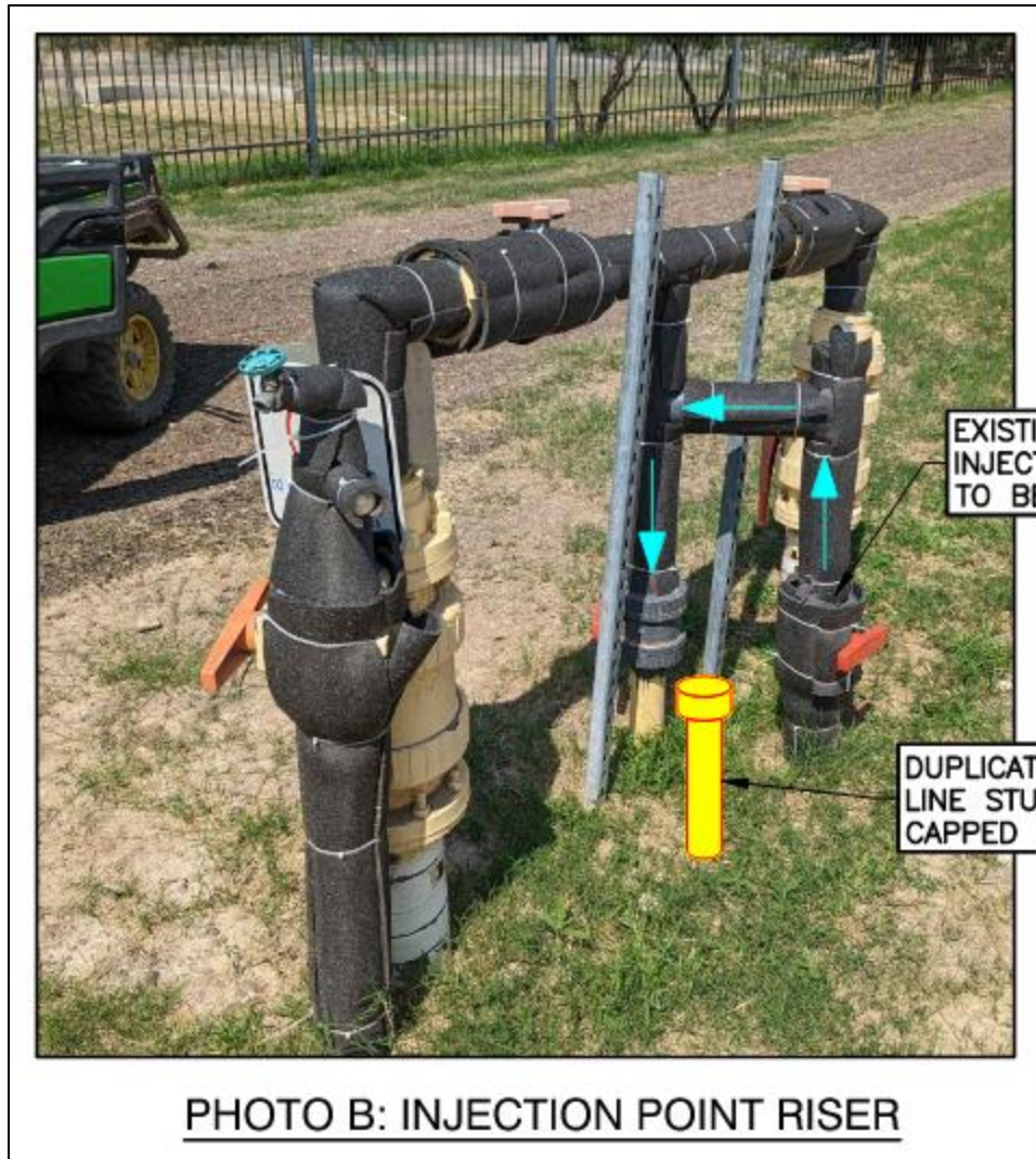
Photo 7 : Excerpt from Drawing Package Showing Piping At Raw Water Injection with Insulation Pre-Construction
