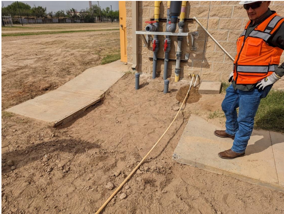
Photo 8: Contractor to replace sidewalk pavement at chemical building that was removed during construction (Refer to punch list item 4)
