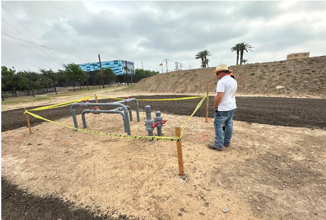
Photo 3 : 3" Tee and reducer location, south view. (Refer to punch list item 3)
