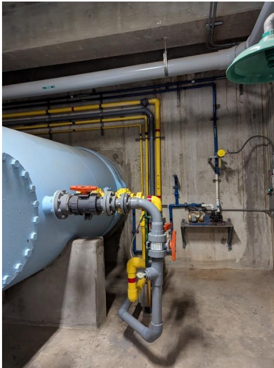
Photos 13 and 14: Contractor to provide labels/stickers for chemical piping inside filter building to City for placement. (Refer to punch list item 5)
