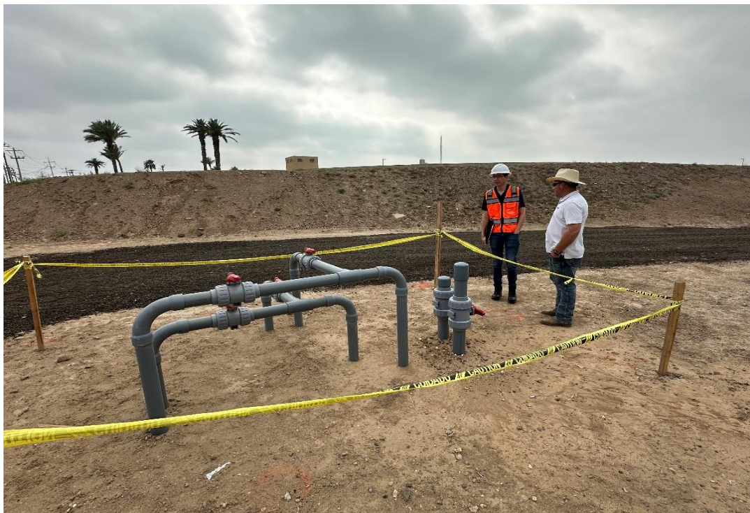
Photo 4 : 3" Tee and reducer location, north view. (Refer to punch list item 3)
