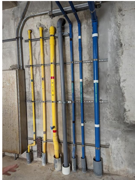
Photos 13 and 14: Contractor to provide labels/stickers for chemical piping inside filter building to City for placement. (Refer to punch list item 5)
